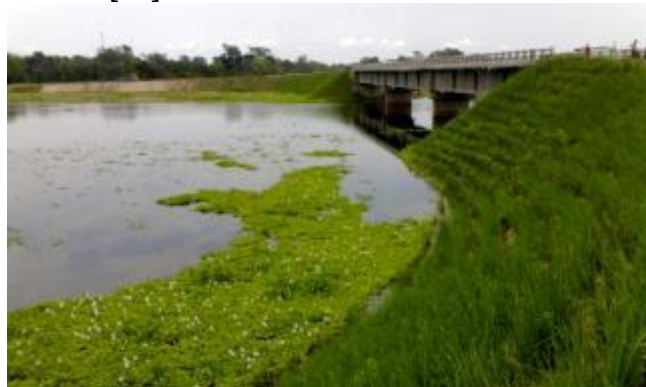
Figure 6. Vetiver Grass on Road Embankment Slopes
